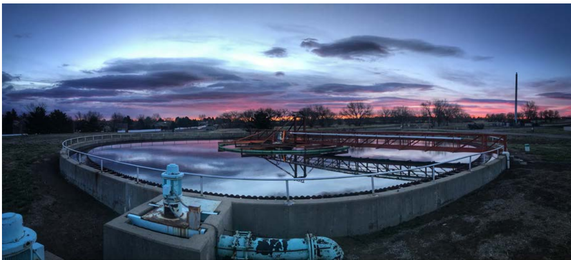
Clarifier at the Water Treatment Facility
